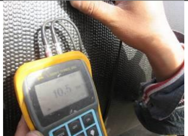
Wall thickness check
